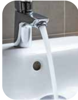
Sinks and taps
